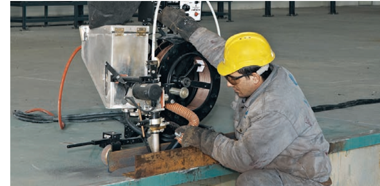
Submerged welding machines
